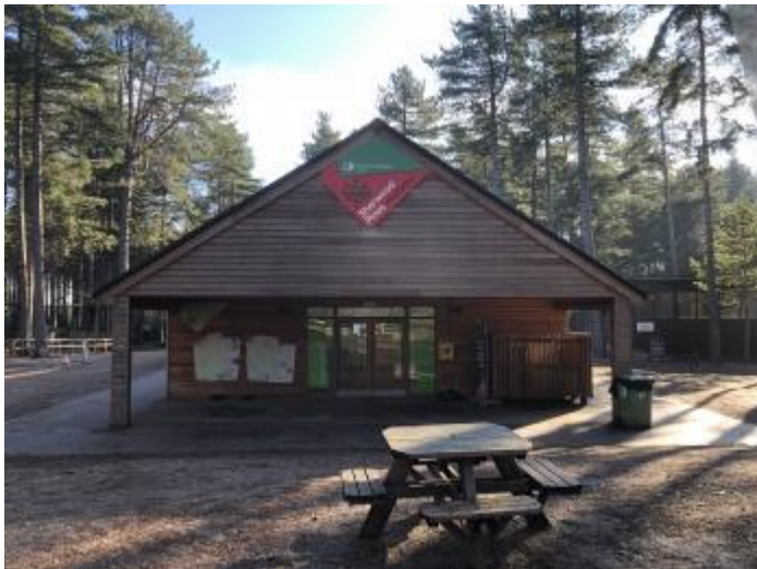
Visitor Centre (Front)
